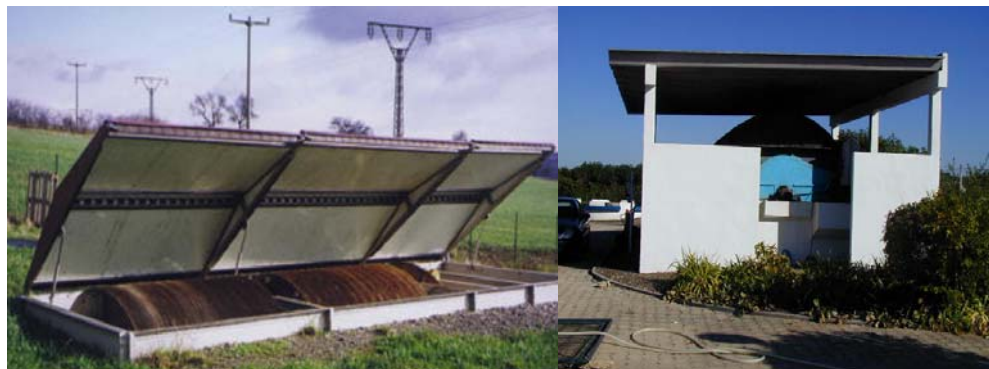
Fig. 8 – Biodisks enclosed and assembled in a building
