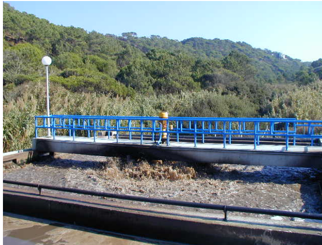
Fig. 10 – Activated sludge aerobic tank (in Magoito Plant)
