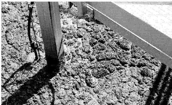
c) foam on secondary clarifier consisting of floating sludge covered bubbles ( d=0.5-2.0\text{mm} ), the color is light brown, but appears white on the picture due to the flashlight
